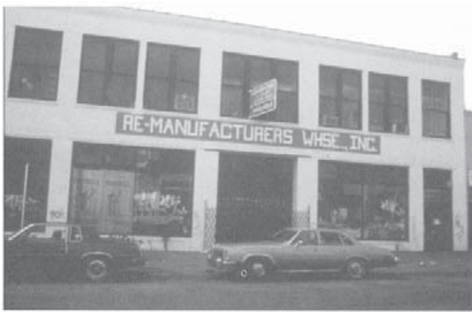
Fig. 14. The site of the new Fairmount Health Center chosen by Jose Galura was an old auto dealership that was converted to a “re-manufacturing” warehouse situated on contested turf between Hispanic and African American communities.
